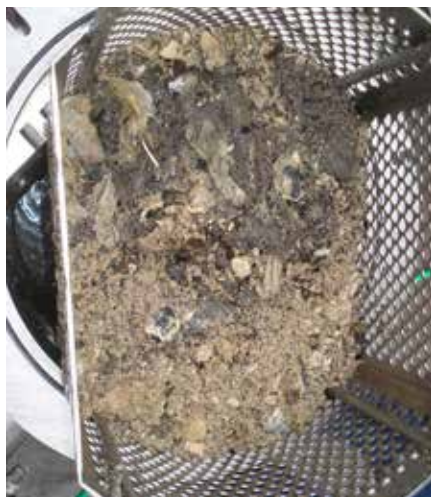
Left: Grease truck unloads using the HOT. Right: The HOT successfully prevents blockage and severe damage that could be done to pumps downstream.
