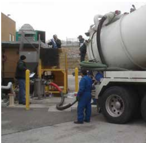
Left: Grease truck unloads using the HOT. Right: The HOT successfully prevents blockage and severe damage that could be done to pumps downstream.
