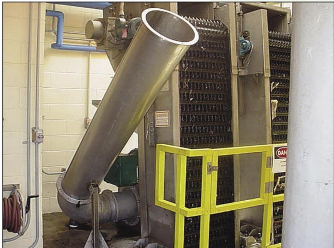
*Clean, compacted screenings discharge is conveyed out the exit chute into a trash receptacle for easy disposal.*
