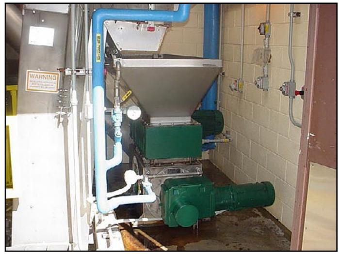
*Screenings from the channel fall into the SWM for washing, compacting and dewatering.*
