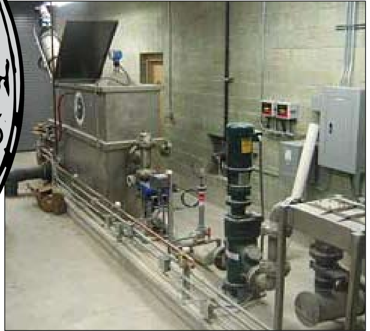
Honey Monster septage receiving station at Smiths Creek Landfill, MI.
