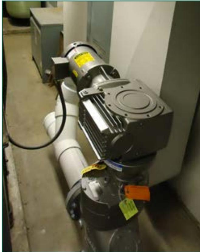
***Thanks to the second of two Monster sewage grinders, there are no more clogged pipelines or pumps wreaking havoc for city engineers.***
