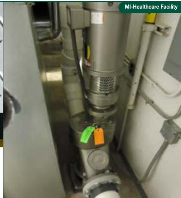
*One of two HYDRO sewage grinders were placed in the basement of this healthcare facility to help reduce clogging.*
