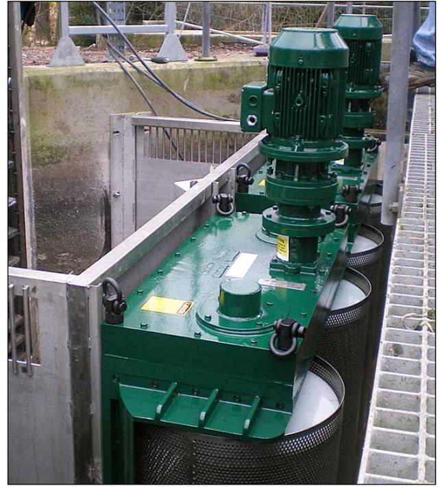
*The Channel Monster combines rotating screening drums with proven Muffin Monster grinding technology.*
