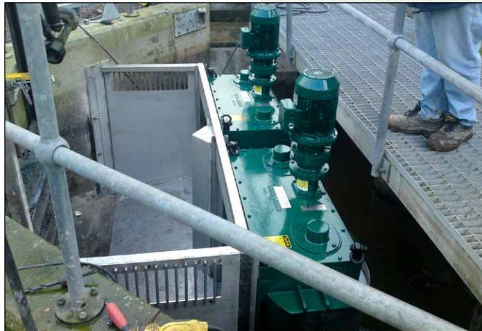
*Shown here are JWCE’s custom made stainless steel inlet channel, overflow outlets with two Channel Monster grinders*
