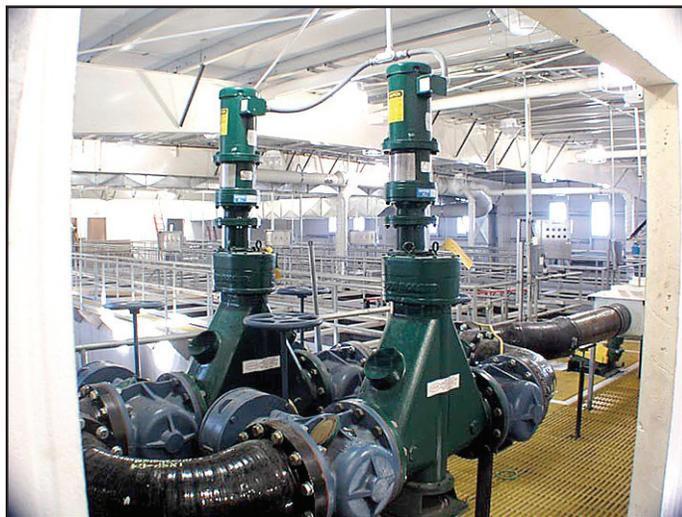
*A pair of Muffin Monsters grind influent entering the McMurdo Research Station wastewater treatment plant, built in 2003.*
