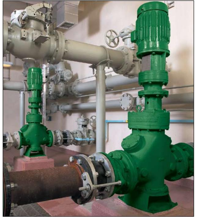
*A pair of Muffin Monsters® are positioned in front of the transfer pumps and grind rags, solids and trash into small particles so they flow harmlessly through pumps and pipes.*
