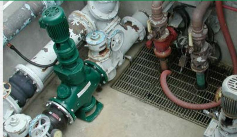
retrofitted into the system ahead of the pumps to shred debris before it creates a clog.
