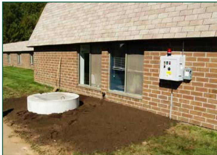
**A Monster 3-HYDRO sewage grinder was installed inside a manhole outside the facility to shred sewage flowing into the city's system.**
