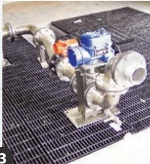
3 The controller activates the Muffin Monster grinder, plug valve\* and flow meter\*.
