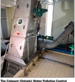
The Cobourg (Ontario) Water Pollution Control Facility installed a 6-mm finescreen with a compactor–washer with only 12 in. (300 mm) to spare in the headworks. Even though the screen catches more trash and debris — preventing it from affecting other treatment processes — the plant now discharges 75% less screenings by volume.
