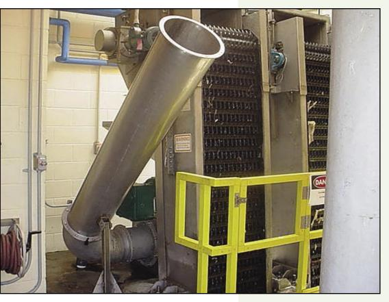
Clean, compacted screenings discharge is conveyed out the exit chute into a trash receptacle for easy disposal.
