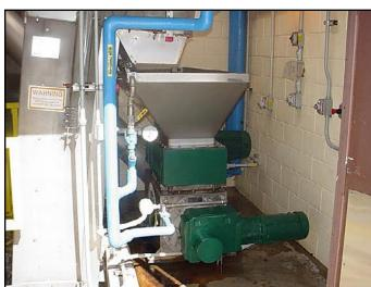
Screenings from the channel fall into the SWM for washing, compacting and dewatering.
