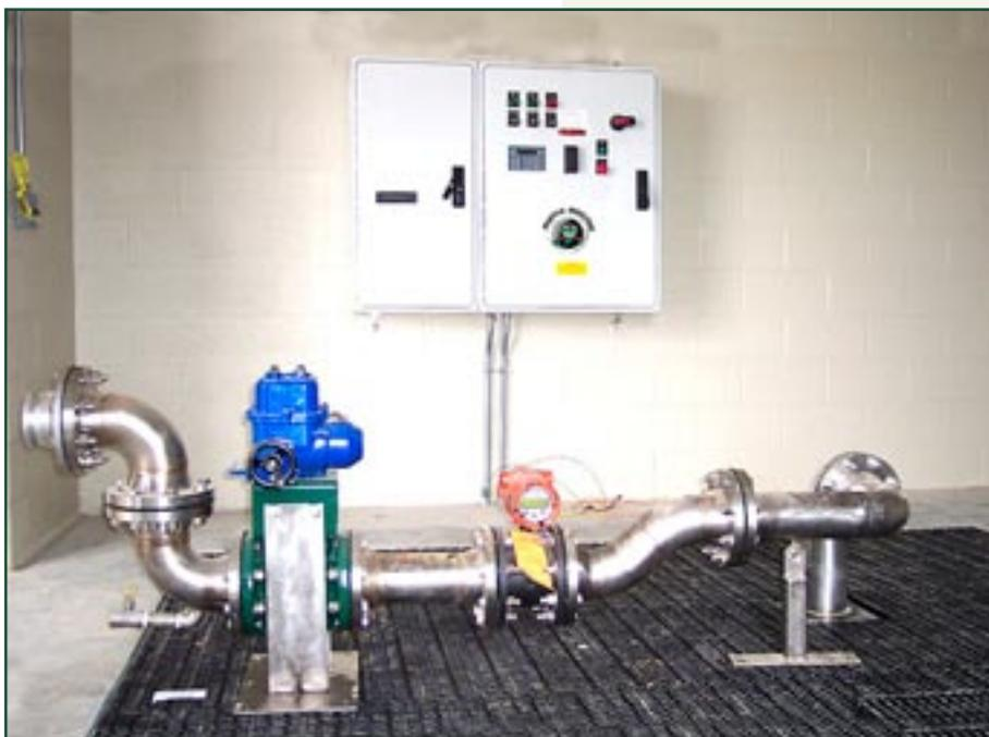
***Here, the Monster Airport Receiving Station is set-up, ready to connect to the airport tugs and quickly remove blue water unloaded from incoming airplanes.***
