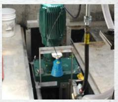
An immersible motor powers an Auger Monster<sup>®</sup> in an underground vault.
