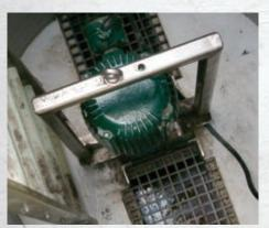
A Muffin Monster<sup>®</sup> with immersible motor and lifting bail in a deep wet well.
