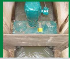
An immersible motor installed on a Channel Monster<sup>®</sup> in a deep channel.
