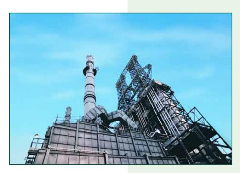
At the Suncor oil sands plant, bitumen is heated and sent to drums where petroleum coke, the heavy bottom material, is removed. Petroleum coke, similar to coal, is used as a fuel source for utility plants.
