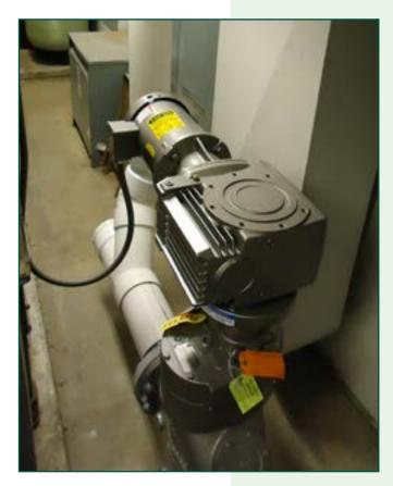
Thanks to the second of two Monster sewage grinders, there are no more clogged pipelines or pumps wreaking havoc for city engineers.
