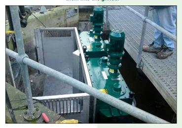
Shown here are JWCE's custom made stainless steel inlet channel, overflow outlets with two Channel Monster grinders
