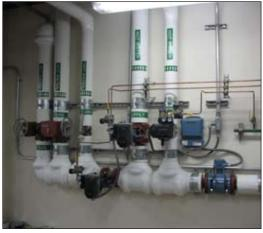
The new biogas-heated hot water loop has ancillary branches to heat the building, front walkway, and headworks washwater.
