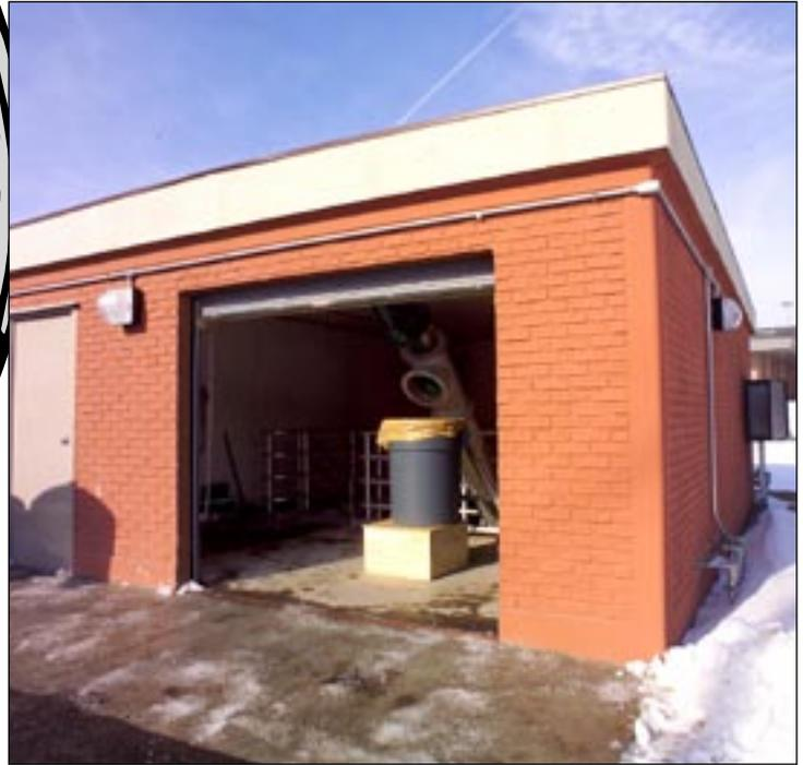
*One of two screening buildings on a large government complex. Inside, an Auger Monster® removes rags and trash from wastewater.*
