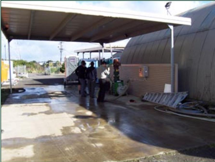
***Operators inspect the Macho Monster, which grinds solids and septage unloaded from their trucks.***
