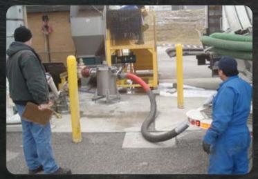
A grease truck unloads through the Monster Industrial Heavy Object Trap and into a wastewater treatment plant's holding tank.
