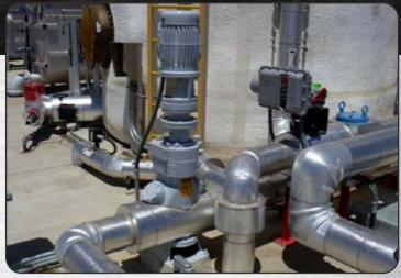
A 3-HYDRO in-line grinder in a grease receiving line.
