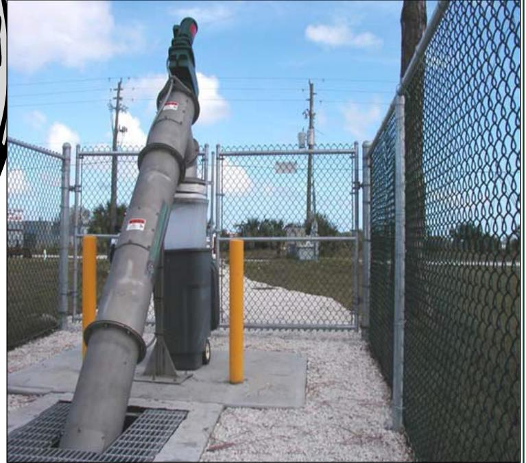
*What goes up...must be bagged! This Auger Monster is located at a County correctional facility where it removes solids from wastewater entering the municipal system.*
