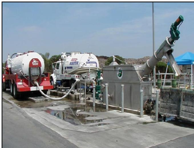
*Emptying septage delivery truck tanks is cleaner, faster, and easier through pipes that connect directly to the SRS.*
