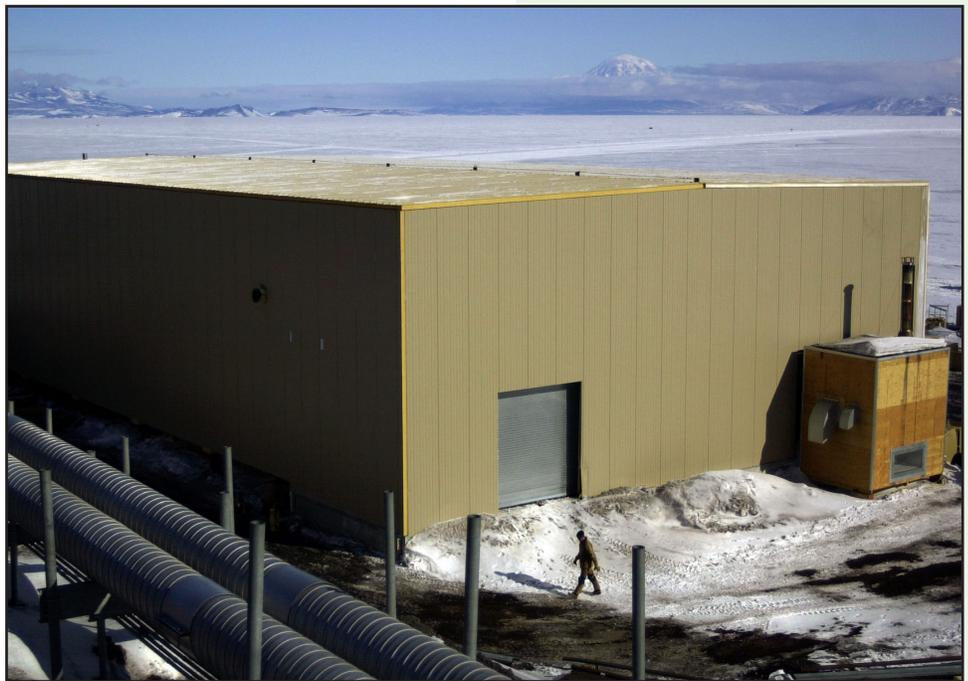
***McMurdo's wastewater treatment plant is housed in a heated warehouse so the treatment process can continue year round.***
