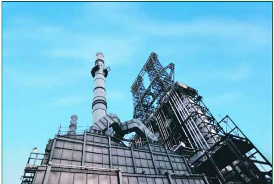
***At the Suncor oil sands plant, bitumen is heated and sent to drums where petroleum coke, the heavy bottom material, is removed. Petroleum coke, similar to coal, is used as a fuel source for utility plants.***
