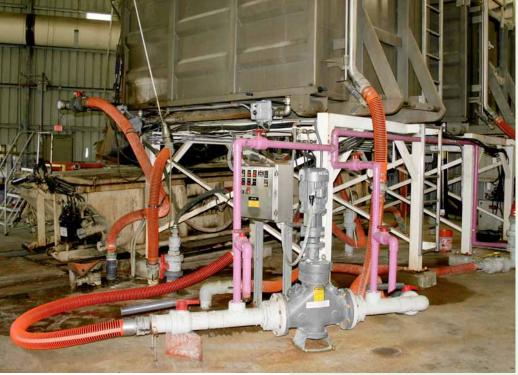
Thickened grease continuously circulates through the 3-HYDRO-IX ensuring the downstream equipment is protected from any foreign material.
