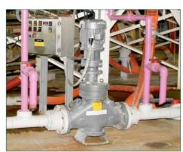
The raw trap grease is chewed up by the 3-HYDRO-IX before entering the storage tank.
