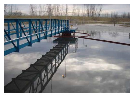
Clarifier mechanisms were replaced, and aluminum covers were installed above the clarifier launders as part of the odor control system.
