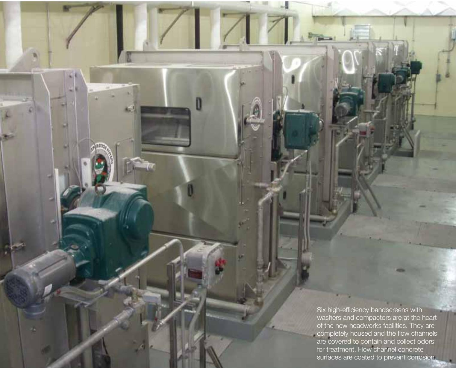
Six high-efficiency bandscreens with washers and compactors are at the heart of the new headworks facilities. They are completely housed and the flow channels are covered to contain and collect odors for treatment. Flow channel concrete surfaces are coated to prevent corrosion.
