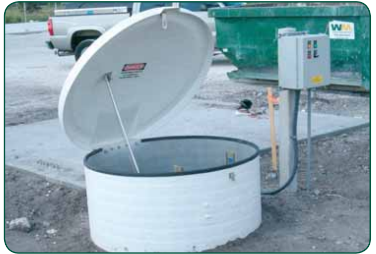
Hatch access door to M3 (street manhole option also available)
