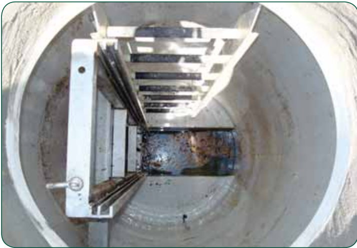
Guide frame and access ladder inside an M3 (the grinder has been removed)
