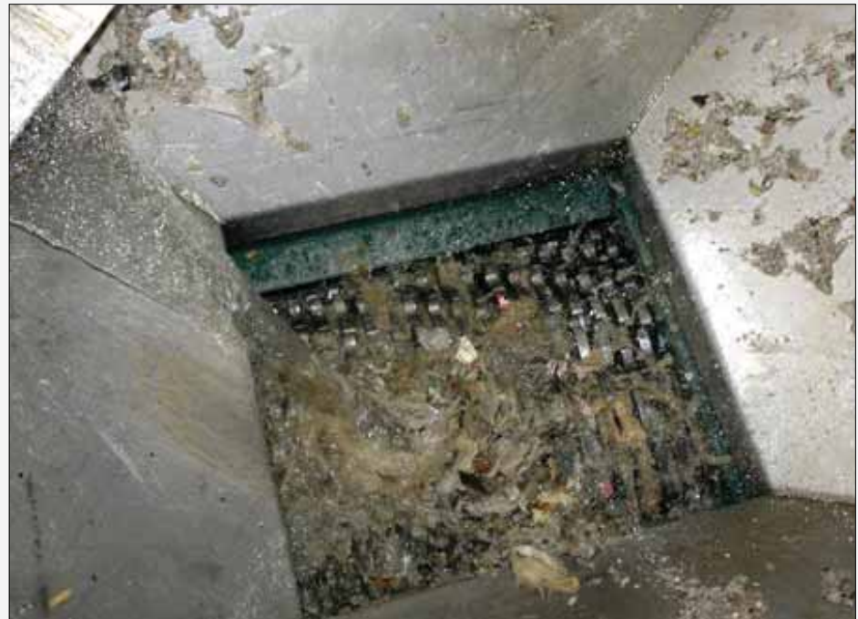
JWC Screenings Washer Monster Hopper View
