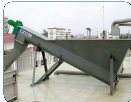
The grit washer and classifier, the last stage in the Grit Monster system.
