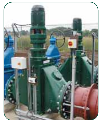
Macho Monster in-line sludge grinders.
