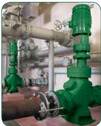
Muffin Monster in-line grinders handling septage.
