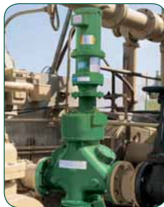
Muffin Monster in-line sludge grinder.
