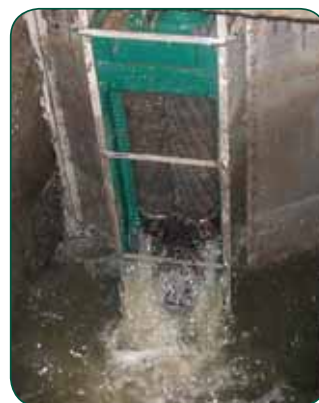
Muffin Monster pump station grinder and installation frame.
