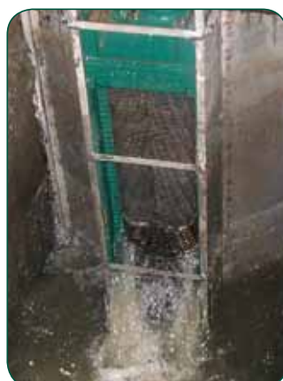
Muffin Monster pump station grinder and installation frame.
