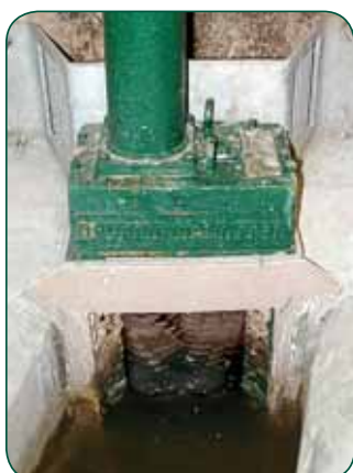
Muffin Monster channel grinder in a prison.
