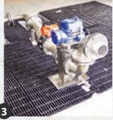
The controller activates the Muffin Monster grinder, plug valve\* and flow meter\*.
